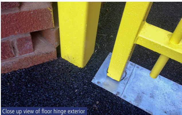
Close up view of floor hinge exterior
