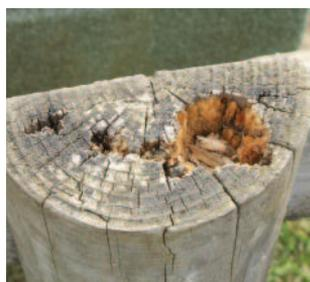
Rotting timber can cause splinters
