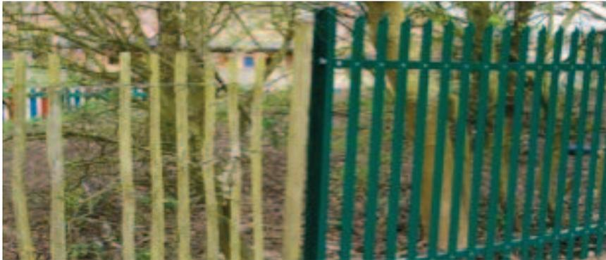
Image shows investment in secure steel fencing which is negated by presence of old timber fencing that is easily penetrable.
