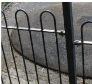
Inadequate spacing between pales, limbs could get trapped
