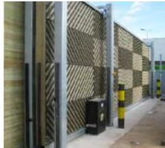
• 4m high x 3m wide acoustic swing and 4m high x 9m wide opening acoustic tracked
