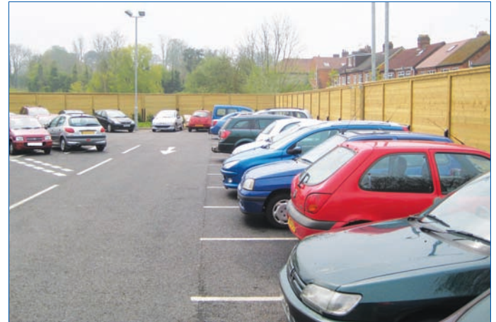
Jakoustic fencing surrounding staff car park
