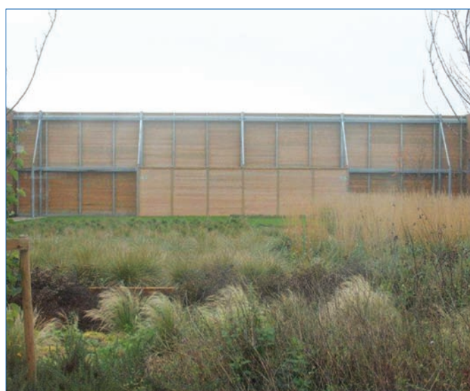
Rear view of the acoustic barrier showing steel frame work
