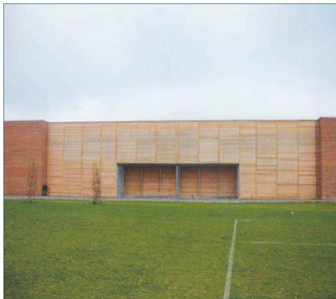
Acoustic barrier constructed from steel posts and acoustic boards
