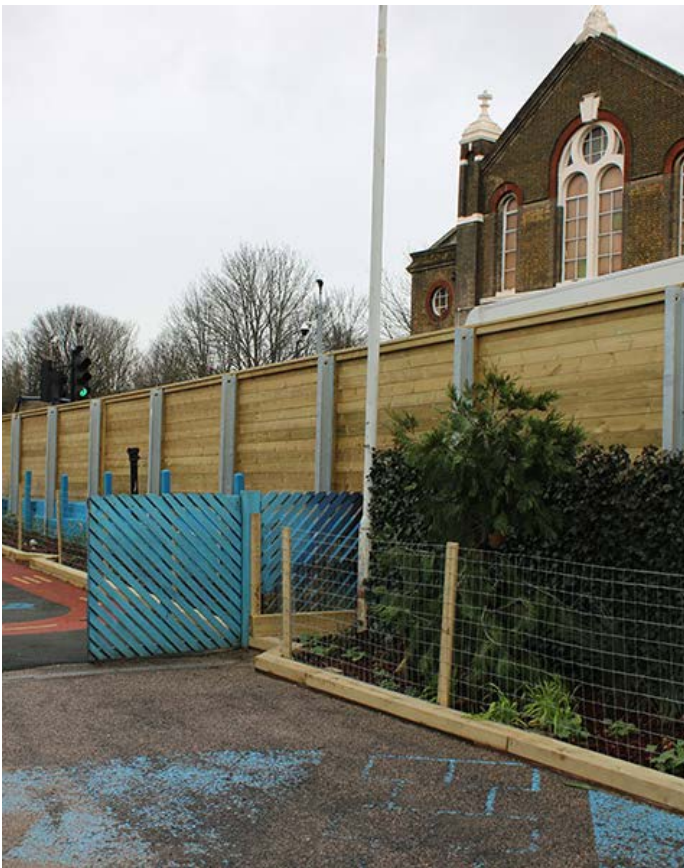
Jakoustic® Reflective barrier with steel I-beams
