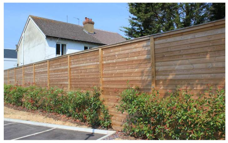
The Jakoustic<sup>®</sup> reflective barrier reflects the noise away using heavy section planed timber boards with a special profile that has been carefully developed. Boards are constructed in such a way that eliminates gaps that sound can easily travel through. Up to 28 dB<sup>\*</sup> in noise reduction.
