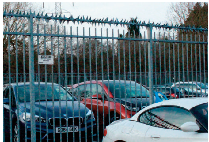
Barbican fencing securing staff car park with Rota Spike® topping
