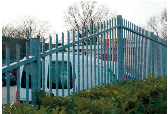
Raked galvanised Barbican fencing
