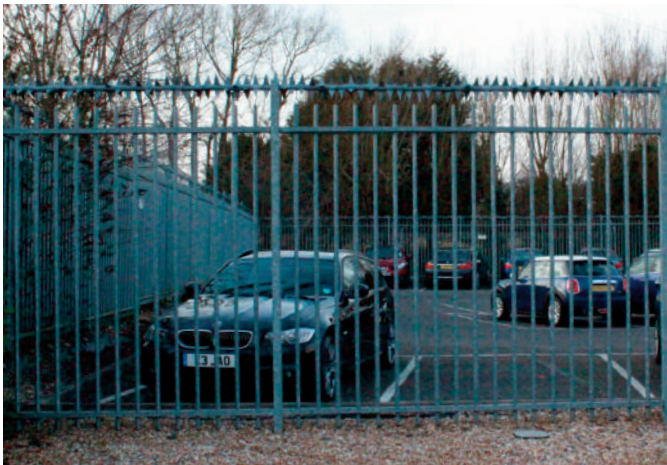
Barbican fencing securing car park with Rota-Spike® topping
