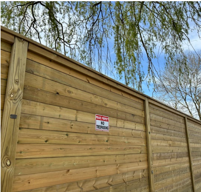
Jakoustic Reflective Acoustic Barrier Detail
