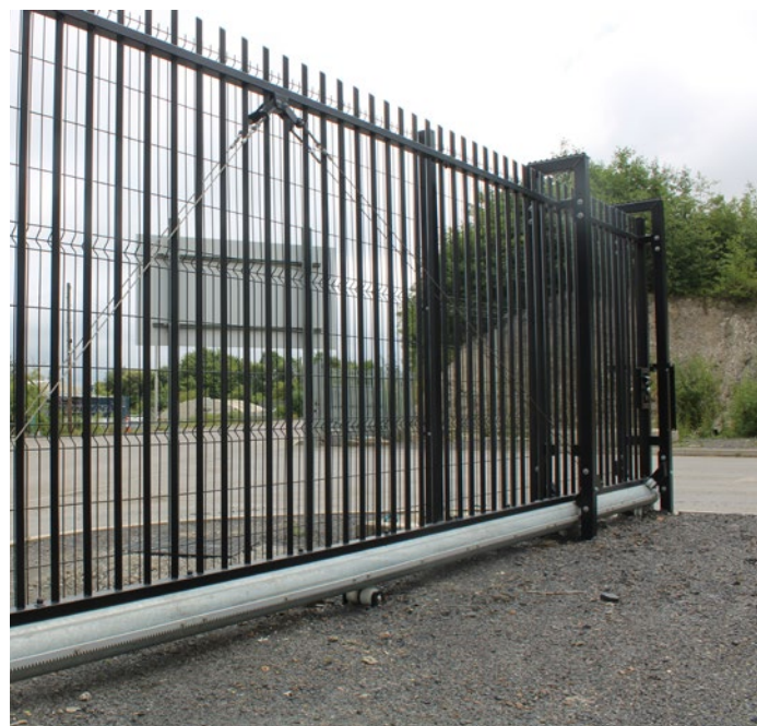
Double leaf Barbican® sliding gate detail
