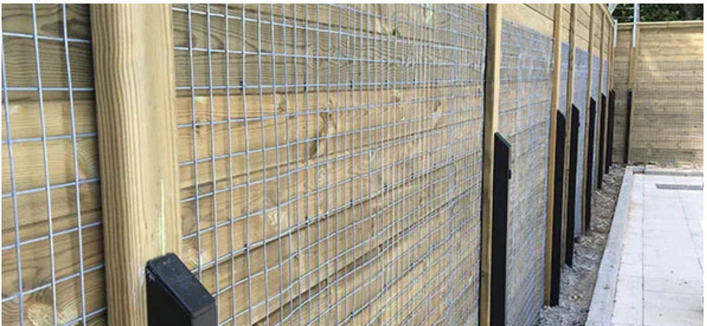
Trident® Jakoustic® acoustic barriers detail
