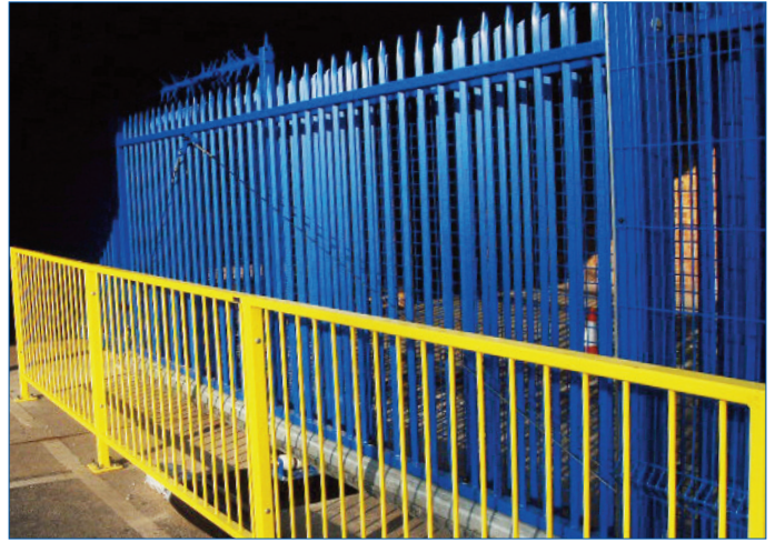
Barbican security railings with Pedestrian Guard Rail
