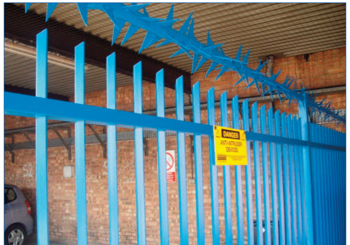
Barbican security railings with security Rota Spike
