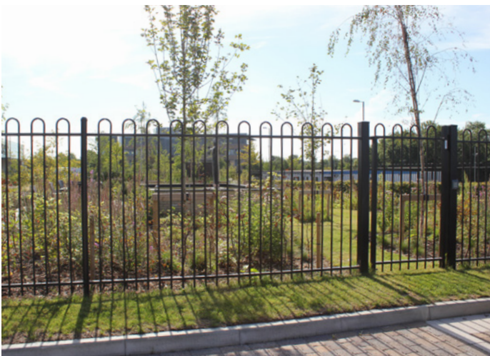
1.8m high Bow Top fencing and gate
