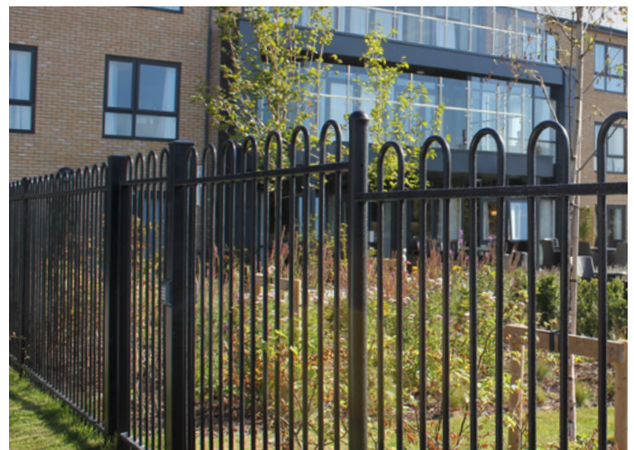
1.8m high Bow Top fencing and gate detail
