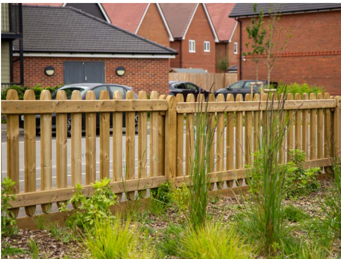
Timber Playtime® fencing around boundary
