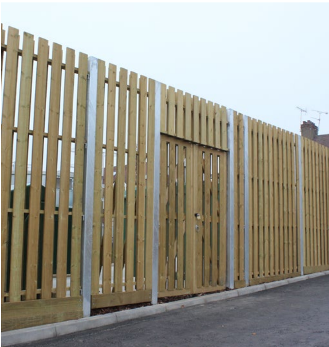
Hit & Miss used to create a secure compound area
