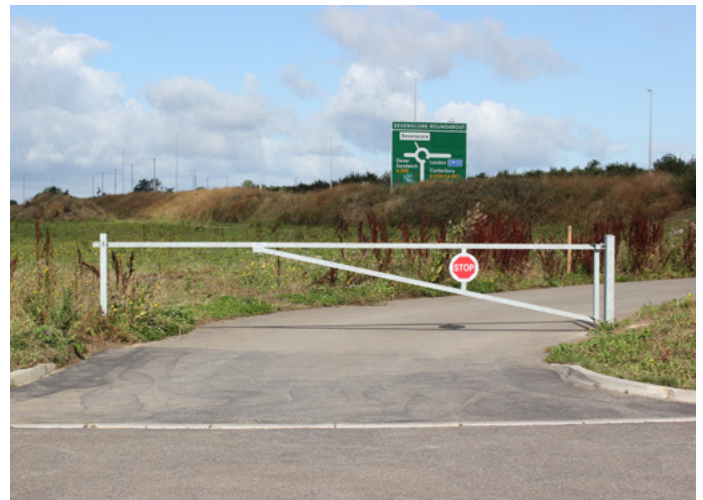
Warden Swing Barrier
