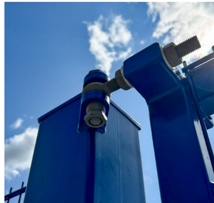
EuroGuard® swing gate hinge detail
