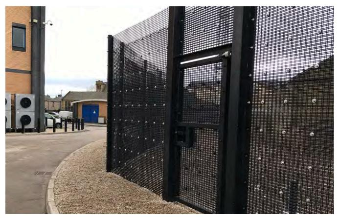
UHS Extreme Mesh SR3 has been designed and tested to withstand forced entry using tools which include battery power tools. The SR3 mesh system is constructed from double skinned mesh providing a high level of security. The fencing and gate system has been developed to meet with demands to give a robust level of security around high security applications.
