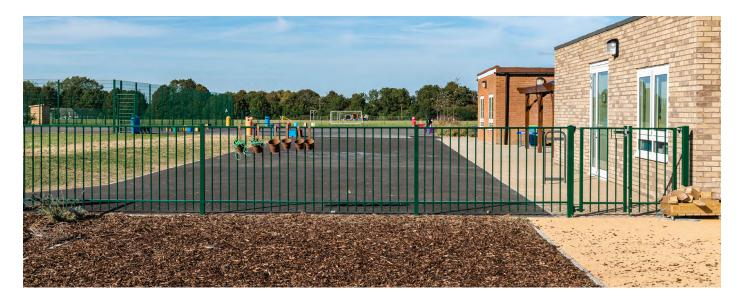
Two-metre tall EuroGuard Flatform Medium was installed around the school perimeter. A matching single leaf gate was installed for pedestrian usage, allowing for better control and monitoring of entry and exit. A manual double leaf gate was installed for vehicular and emergency access.
