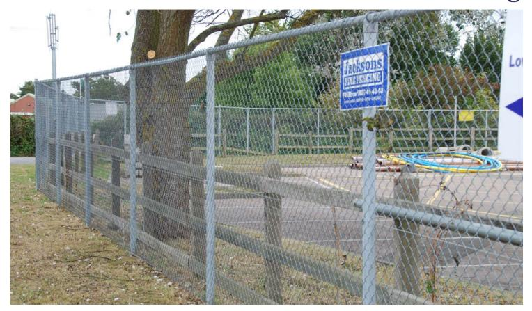
Unlike generic systems, Jacksons Tubular Systems for Chain Link and Welded Mesh fencing can feature a top rail for added security and strength. They are made entirely from steel, galvanised as standard or galvanised and powder coated to BS EN 13438 in one of our standard colours.
