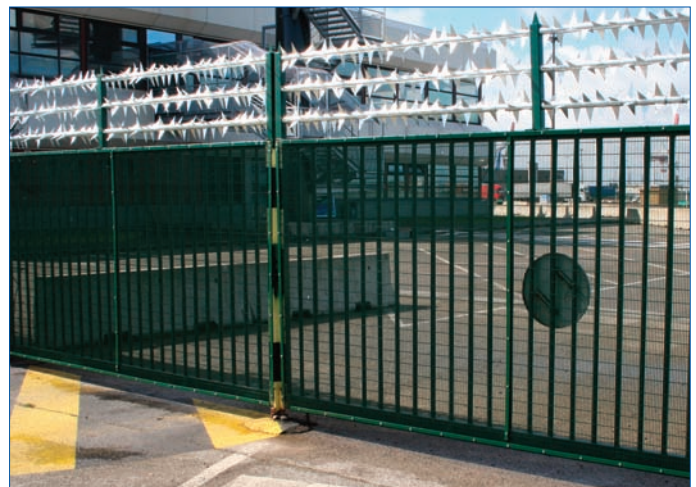
Large manual Sentry gate with Welded Mesh panels and three rows of Rota Spike
