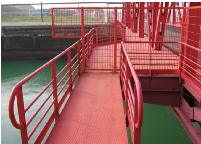
Bespoke steel security panels to match the existing handrail and decking, capable of accommodating the regular lifting of the bridge.
