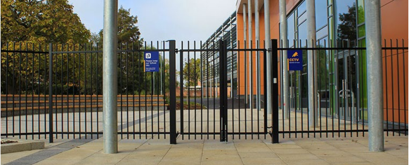
Barbican Imperial® fencing and double-leaf pedestrian gate around the front of the school
