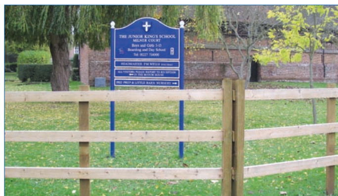
Three rail standard post and rail fencing
