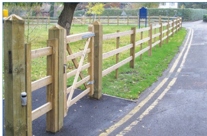
Post and rail fencing with pedestrian uni-gate around the exterior perimeter
