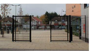
If the gate forms part of an emergency escape route, the release mechanism will need to be of a keyless design and protected to prevent operation from the outside of the gate.
