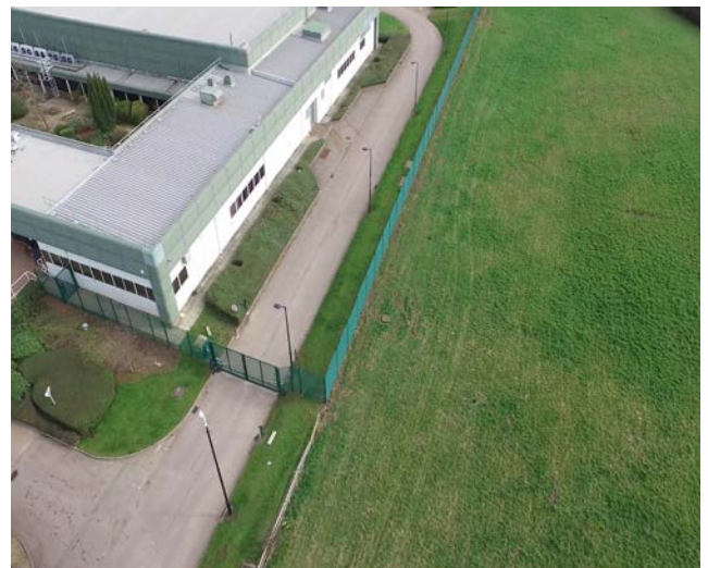
Fencing along the perimeter with double leaf gate for access control
