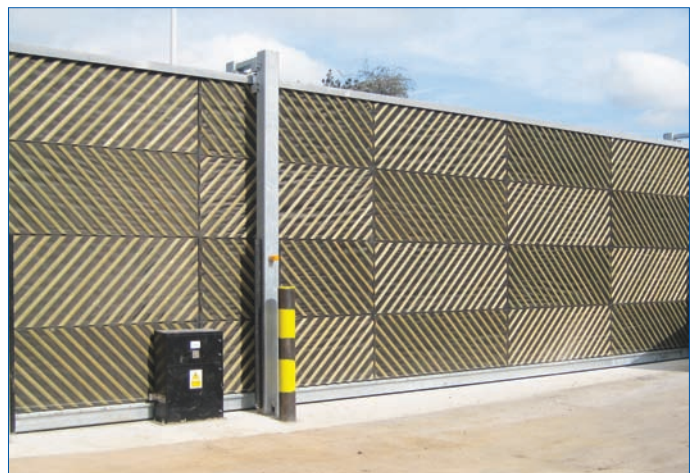
Back of large Jakoustic gate showing absorptive panel detail used
