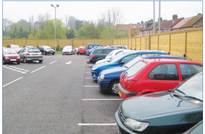
Jakoustic fencing surrounding staff car park
