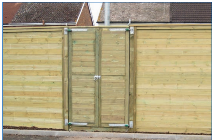
Jakoustic gate for access to lamp post
