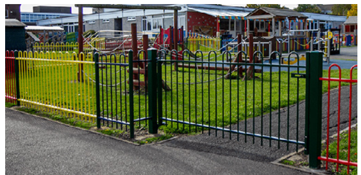
Bow Top Fencing and Gate
