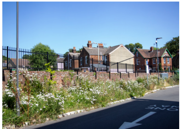
Barbican® fencing on bespoke cranked posts
