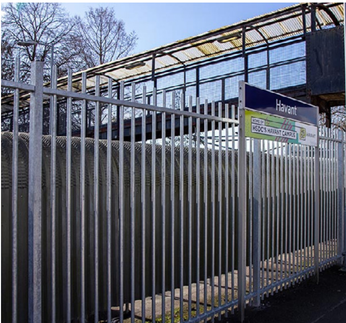
Barbican Imperial® fencing at Havant Station
