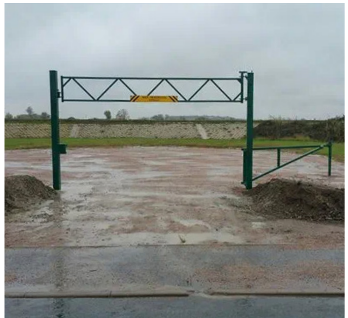
Our max height barrier was installed at Shingle Beach in Sheppey
