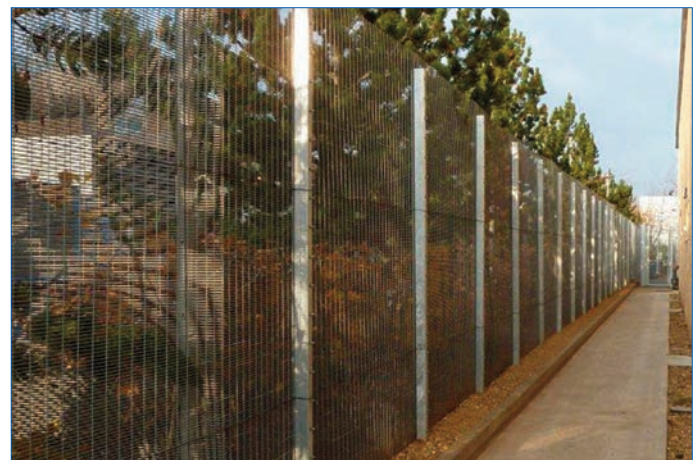
Securi Mesh fence run
