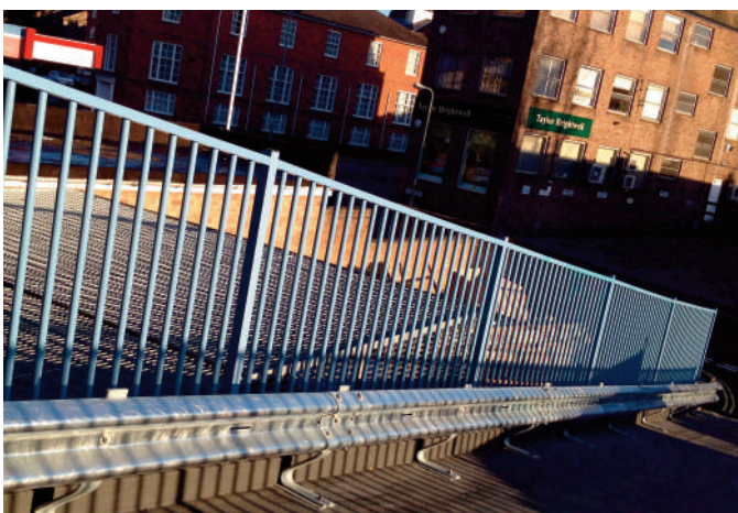
Sentry security fencing with semi pale-through-rail construction
