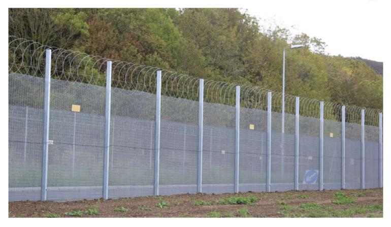
Securi-Mesh<sup>®</sup> Plus features anti climb double layer mesh panels with small apertures to eliminate foot and finger holds, preventing objects being passed through. The system is particularly effective against the use of conventional hand and portable power cutting tools.
