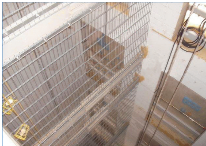
60m lift shaft clad with EuroGuard
