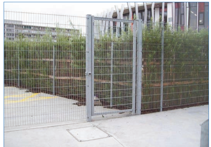
EuroGuard platform fencing and gate
