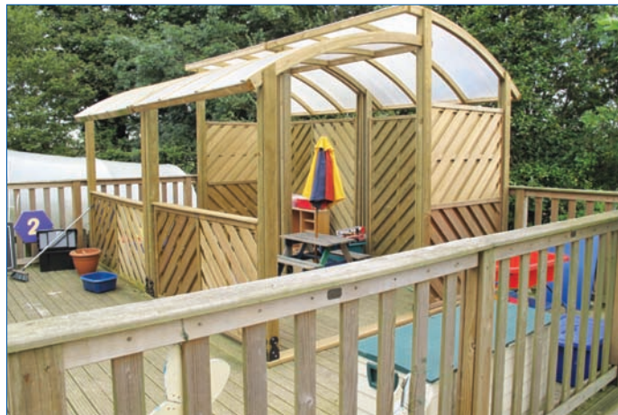
Play area showing balustrade used as a safe perimeter to the decking
