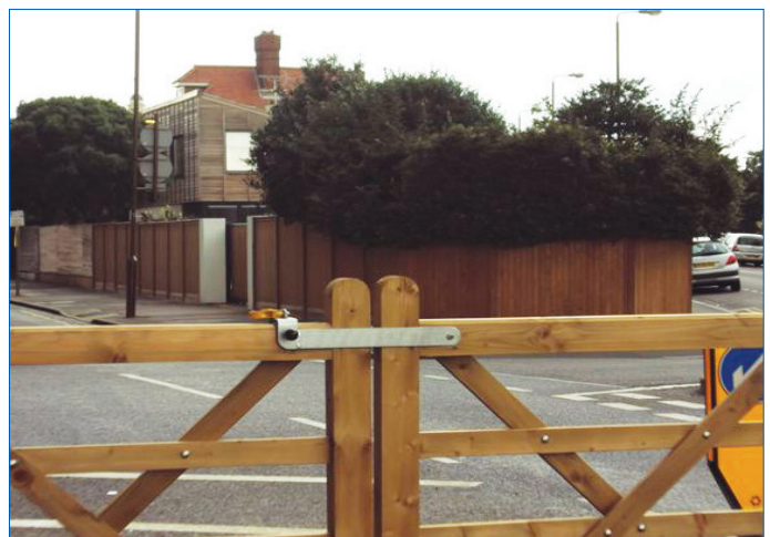
Detail of the gates 'loop over' fittings
