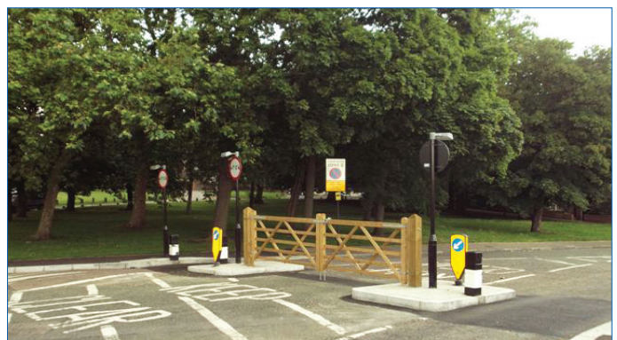
One of the other new emergency gates in situ in Blackheath
