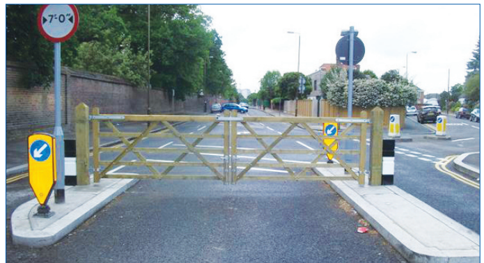
The previous location now with new gates and pinch point upgraded
