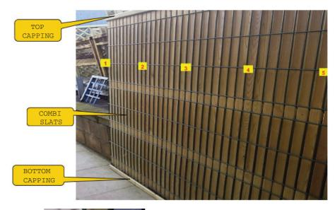
**STEP 2:** Push the BOTTOM CAPPING up against the inserted COMBI SLATS and fix them in place using Screws M4 x 45mm from front side of the EUROGUARD
